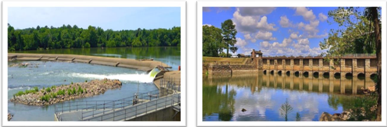
Figure 26. Two Views of Head Gates
