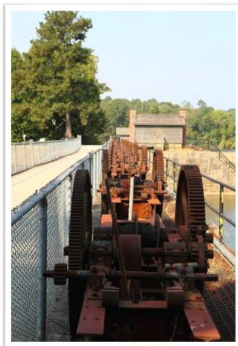
Figure 27. Head Gates Mechanism
